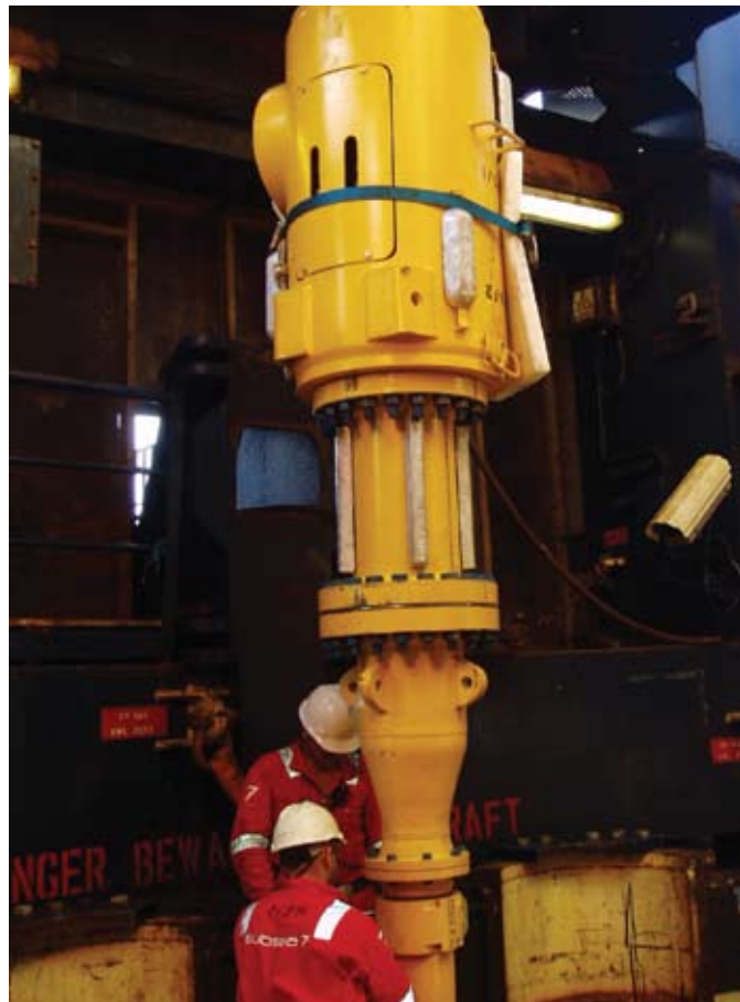
Umbilical installation deployed by the Toisa Perseus
