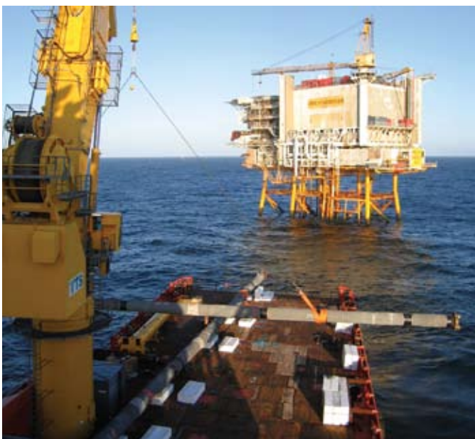
Subsea 7 put seven spool pieces in the bypass around the platform
