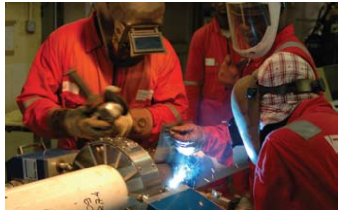
Angolan Welders fabricating flowline stalk at Luanda spoolbase
