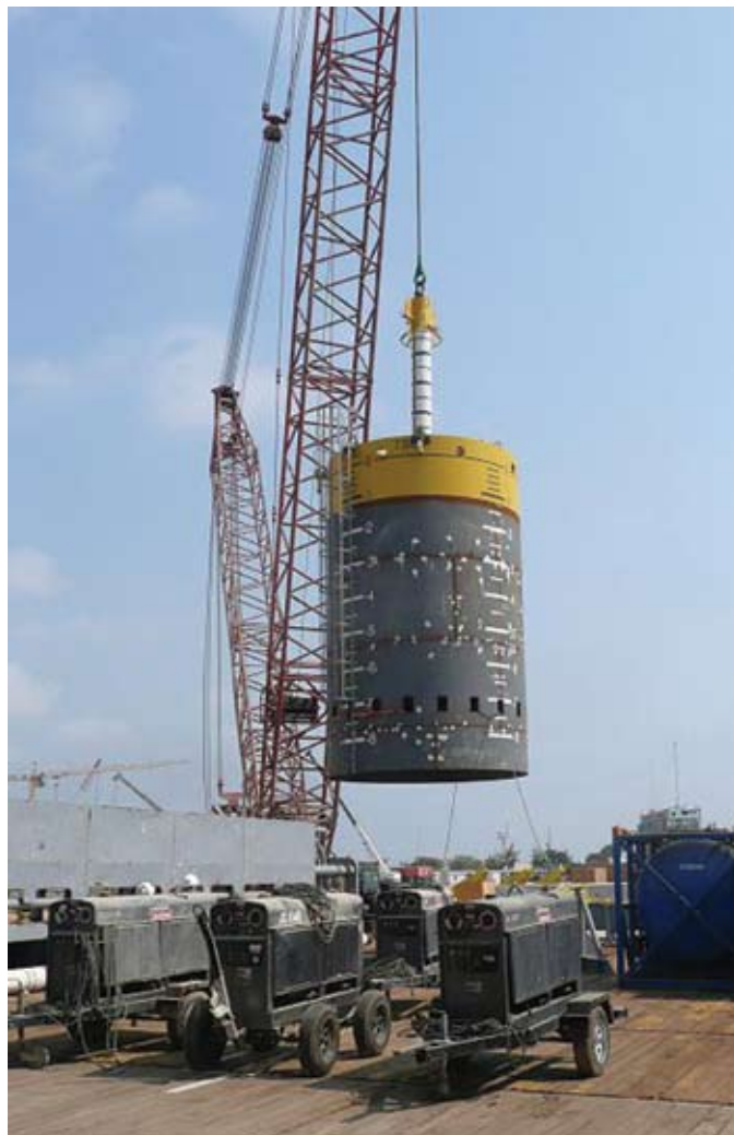
Suction pile for production manifold
