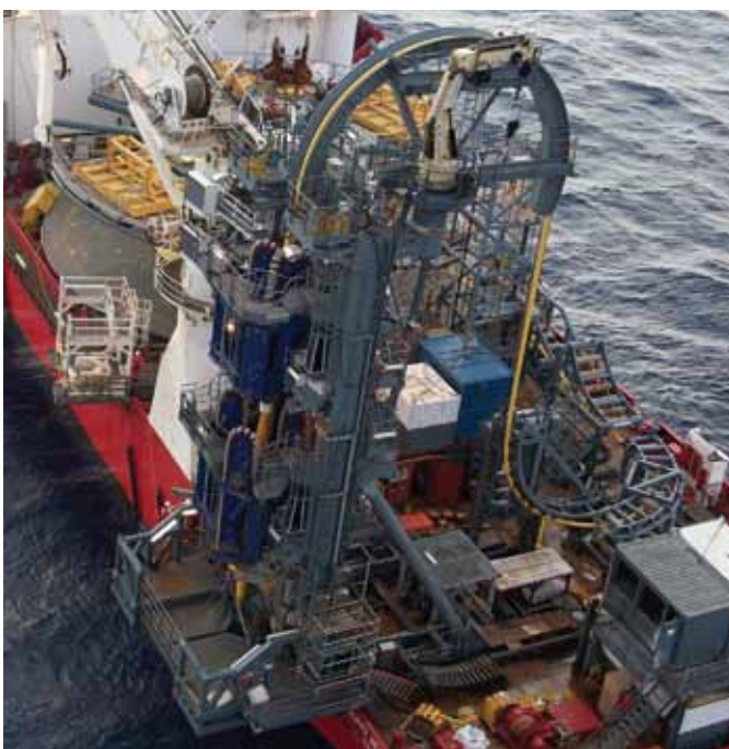
PVLS system in operation
