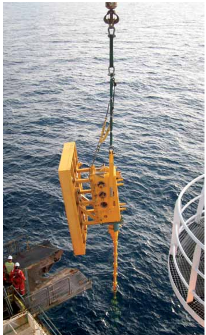
Deployment of Subsea Termination Assembly
