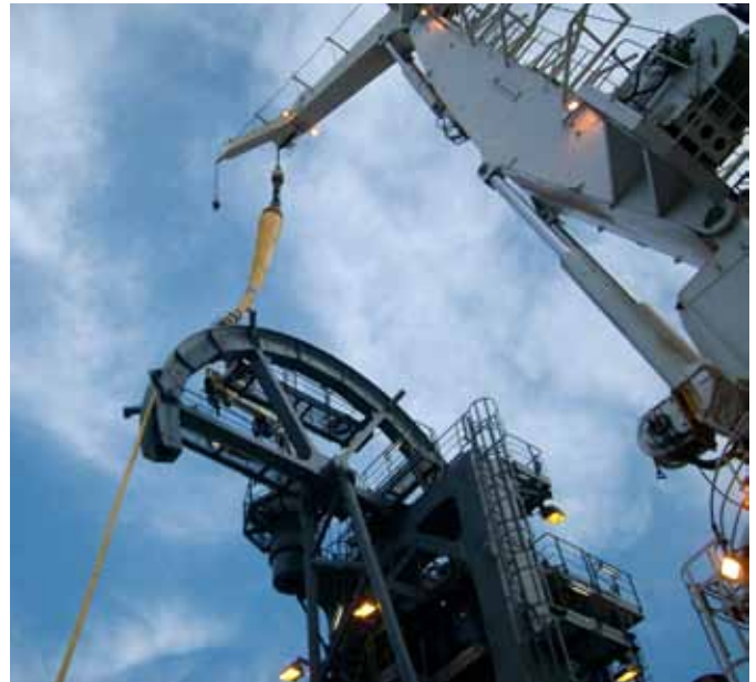
Manoeuvring Bend Stiffener over PVLS
