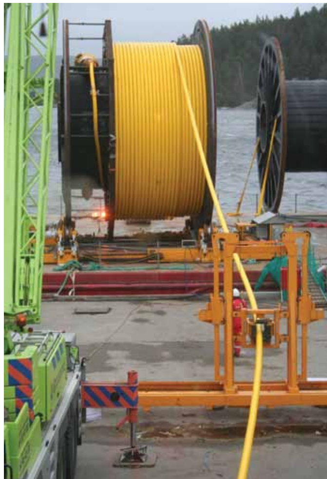
Loadout of umbilical in Norway
