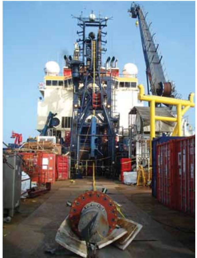
Umbilical installation on the Toisa Perseus
